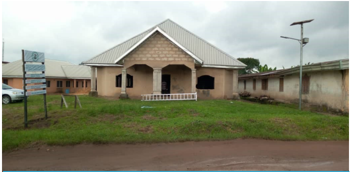
CONSTRUCTION AND COMPLETION OF AGBAMUZU TOWN HALL
