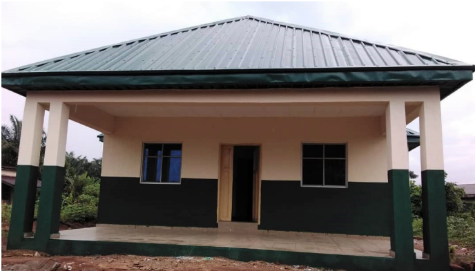
CONSTRUCTION OF MATERNITY HEALTH CENTRE WITH EQUIPMENT IN BENDE
