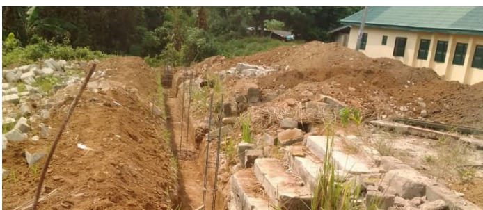
CONSTRUCTION OF UBIBIA CENTRAL SCHOOL NKPORO
