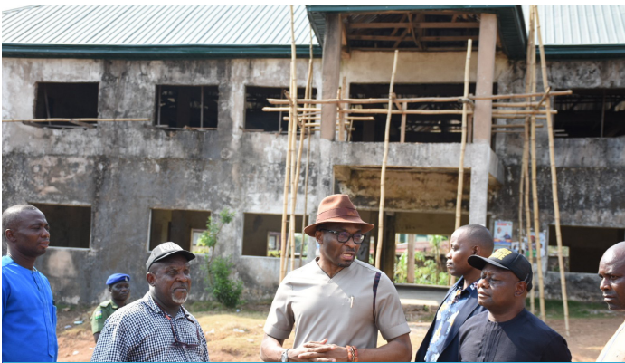
REHABILITATION OF UCHE EBIRI HALL IN IGBERE
