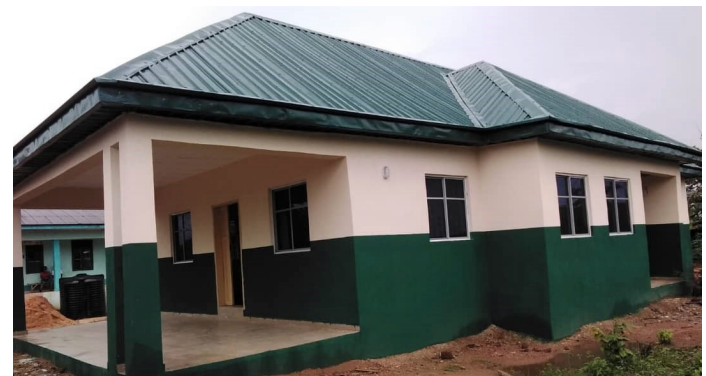
CONSTRUCTION OF MATERNITY HEALTH CENTRE WITH EQUIPMENT IN BENDE
