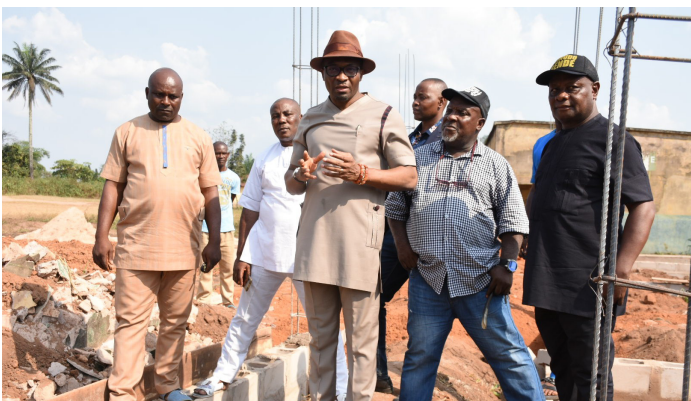
REHABILITATION OF UCHE EBIRI HALL IN IGBERE
