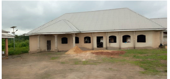
CONSTRUCTION AND COMPLETION OF AGBAMUZU TOWN HALL
