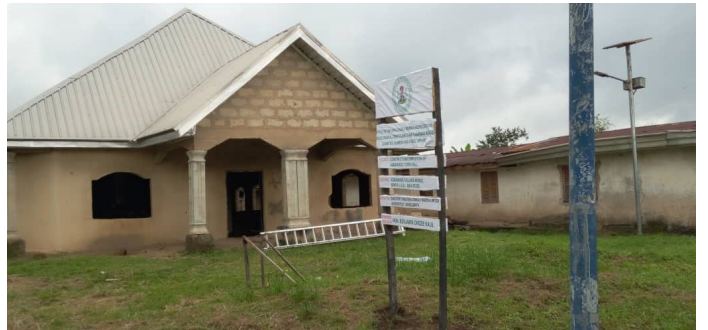
CONSTRUCTION AND COMPLETION OF AGBAMUZU TOWN HALL
