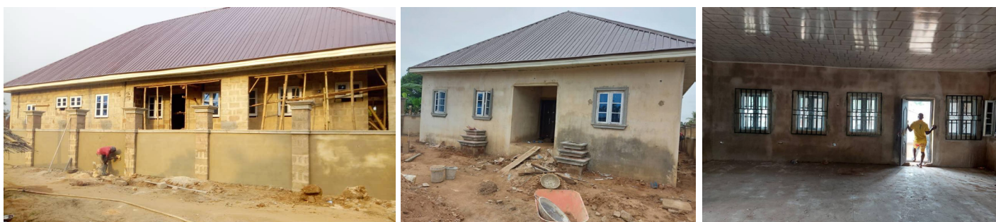
AFTER - NTALAKWU HEALTH CENTRE (UNDERGOING REHABILITATION)
