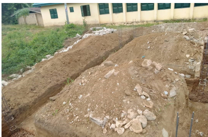
CONSTRUCTION OF UBIBIA CENTRAL SCHOOL NKPORO
