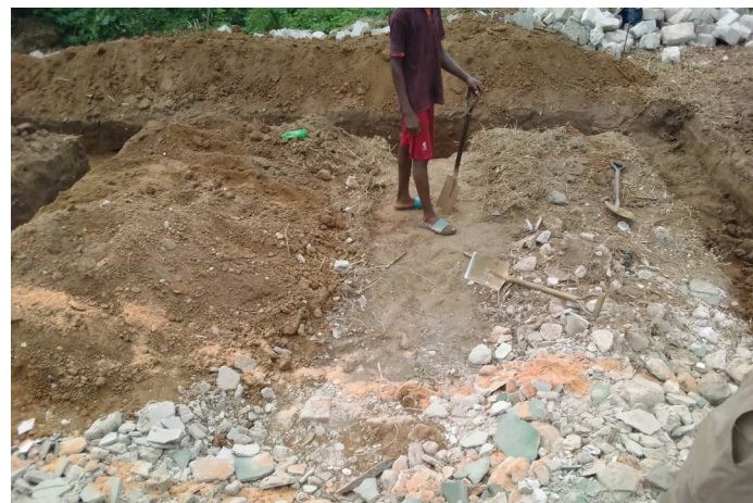
CONSTRUCTION OF UBIBIA CENTRAL SCHOOL NKPORO
