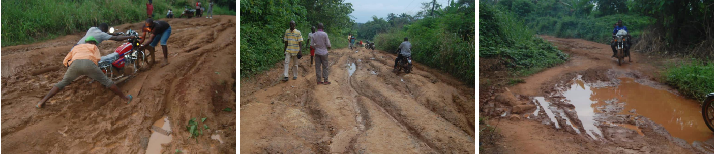
BEFORE - STATE OF THE ETITULO-ITUMBAUZO ROAD BEFORE REHABILITATION
