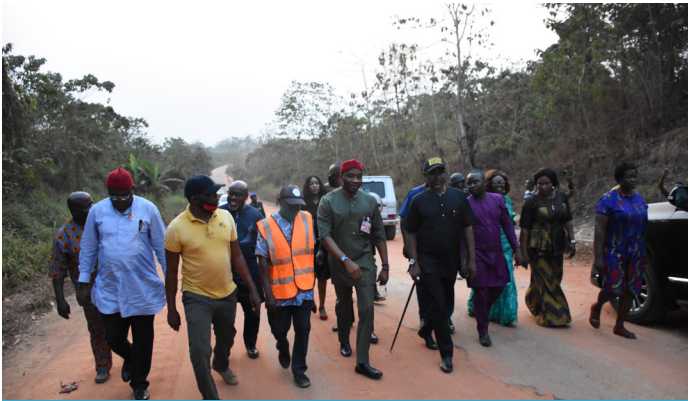
REHABILITATION OF ETITIULO-ITUMBAUZOR ROAD
