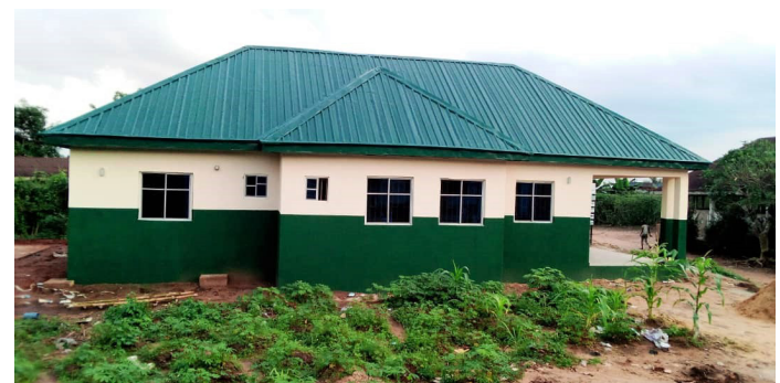
CONSTRUCTION OF MATERNITY HEALTH CENTRE WITH EQUIPMENT IN BENDE
