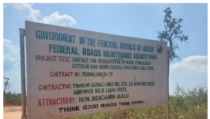
REHABILITATION OF ETTIULO-ITUMBAUZOR ROAD
