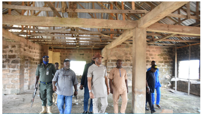
REHABILITATION OF UCHE EBIRI HALL IN IGBERE
