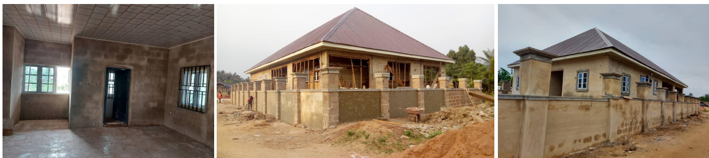
AFTER - NTALAKWU HEALTH CENTRE (UNDERGOING REHABILITATION)
