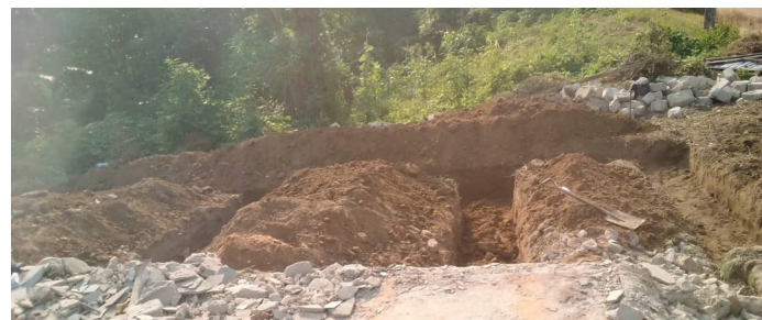
CONSTRUCTION OF UBIBIA CENTRAL SCHOOL NKPORO
