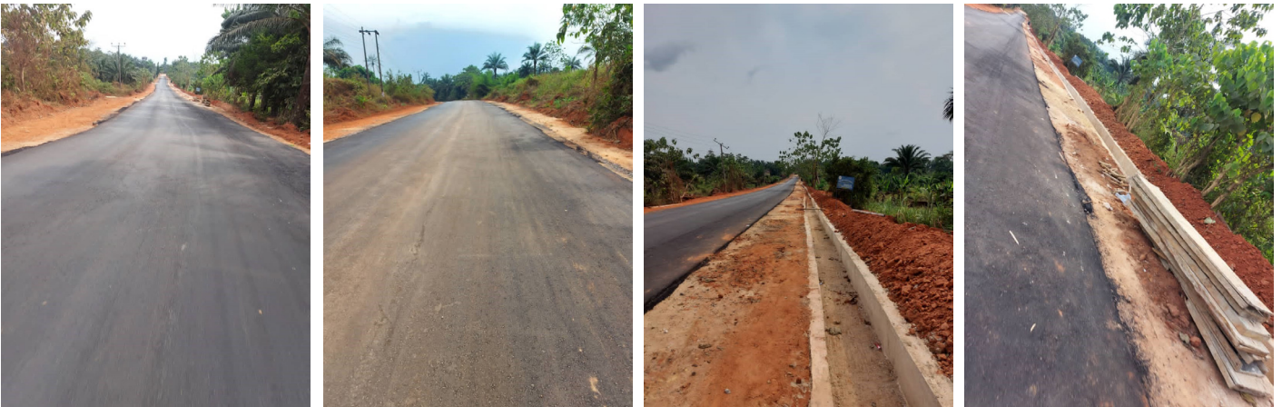
AFTER - STATE OF THE ETITULO-ITUMBAUZO ROAD
